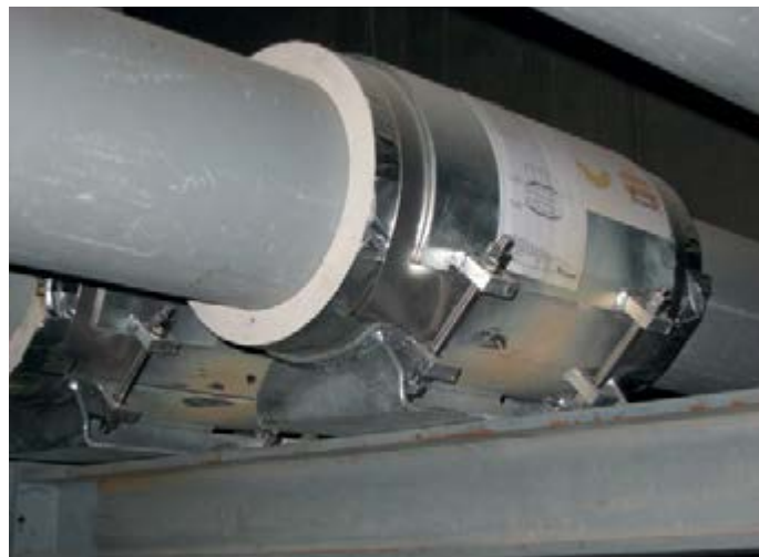
Cryogenic clamp base type 56
