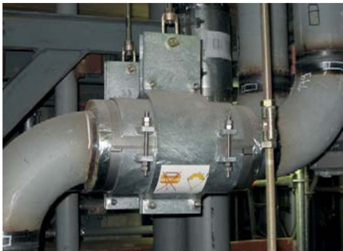
Suspension with cryogenic pipe clamps
